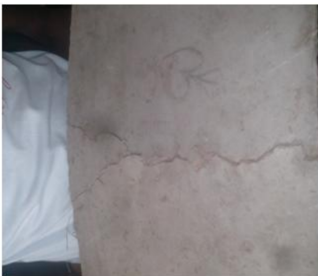
Figure 3.5: Shows the failure state of the Specimen when subjected to flexural bending.
