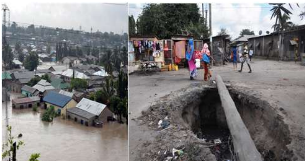
Figure 17: Vulnerable houses at Msimbazi valley Source: Field Survey May, 2016
