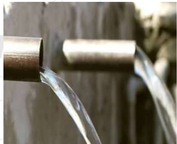
Figure 5: Water entering collection unit
