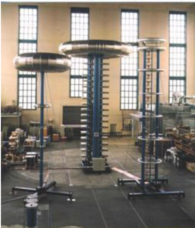
Figure 4: Impulse Voltage Test System IP 360/3600 G (360 kJ, 3600 kV) with impulse voltage divider and chopping multiple spark gaps, with stage energy of 20 kJ being used for the LI test of power transformers up to 765 kV
