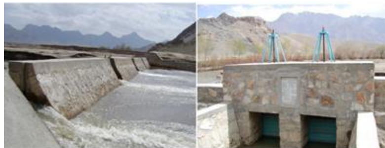
Figure 11: New Dam and Creation of Typical Canal Gate's in the Logar River
