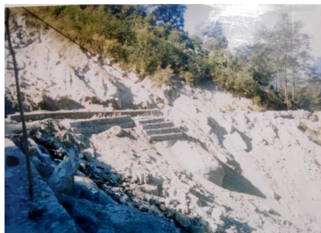
Figure 1: Lantakhola landslide area as viewed in field from northern direction
