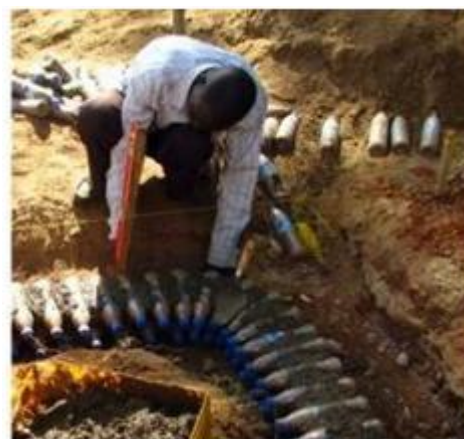
Figure 4 (a): Corners in plastic bottle masonry Image courtesy: building with bottles: an earth day update APRIL 22, 2011
