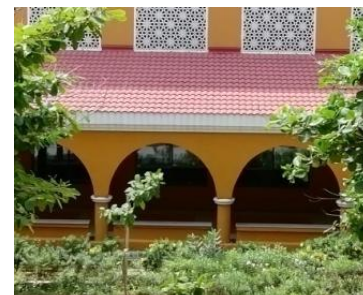
Figure 12: Roof (Source: author)
