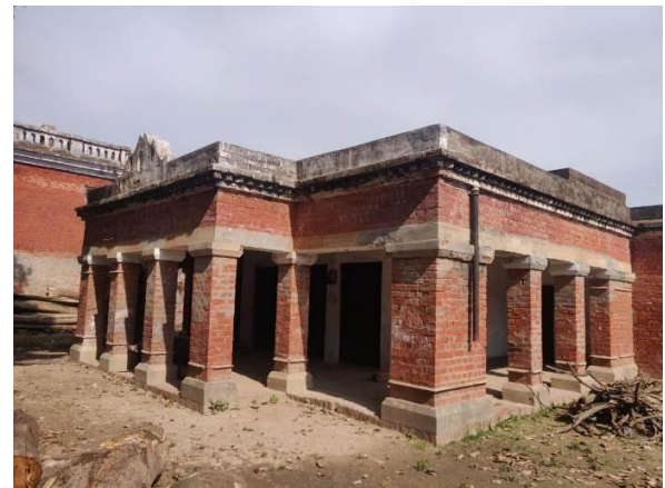
Figure 19: Sona Bai Kothi, Takia Sharif Source (Kant, 2019)
