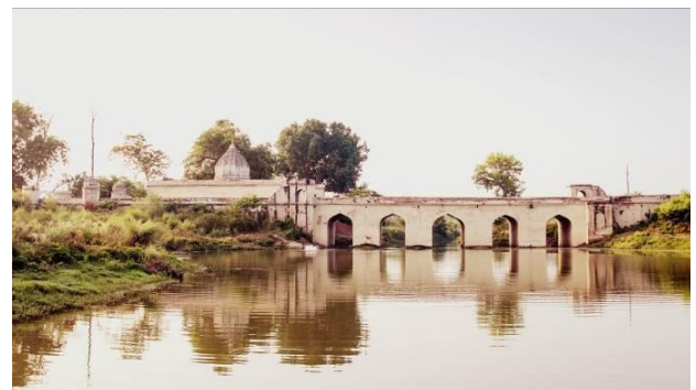
Figure 2: Beheta Bridge and Temples Source:(Kant, 2019)
