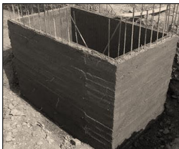
Figure 3: Photographic view of the UG tank at the time of construction
