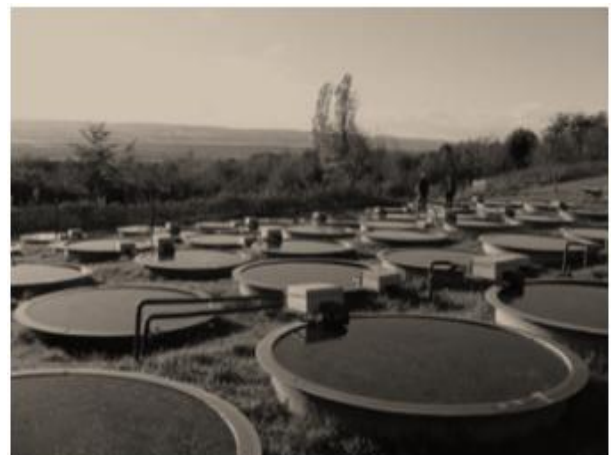
Figure 1: Photographic view of underground water tank
