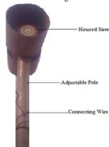
Plate 1: Picture showing the Installed Siren on Pole
