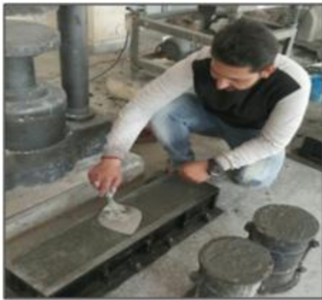
Freshly prepared Beams
