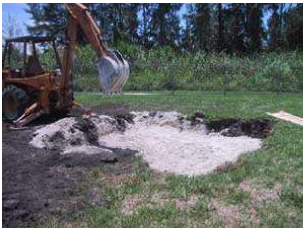
Excavating the whole for the antenna
