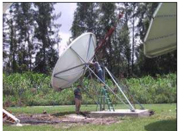
Alignment of the antenna
