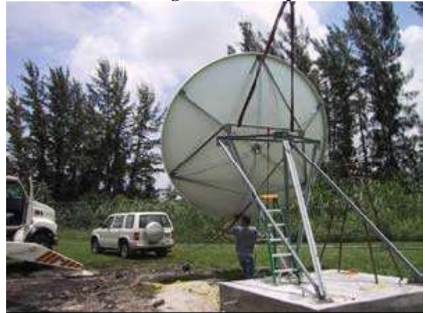
Installing the antenna on the support frame
