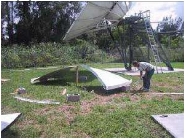
Professional installer begins assembly of an Andrew 4.5m
