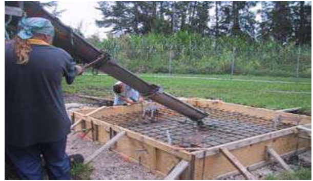
Building the concrete pad
