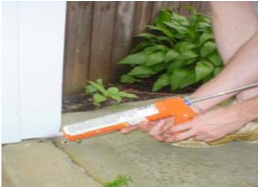
Figure 8: Seal up the hole inside & outside of the home to keep rodents out}
