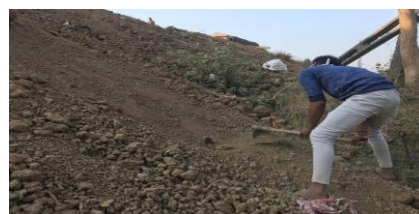
Figure 4: Preparation of site
