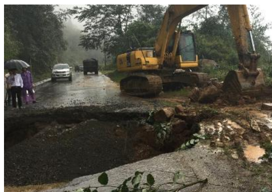
Figure 28: Collapses on Km9+500, related underground karst in Nung Nang commune, Tam Duong district in 2019.
