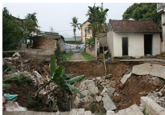
Figure 29: Collapses on My Duc district, Hanoi , Hanoi related underground karst in 2001
