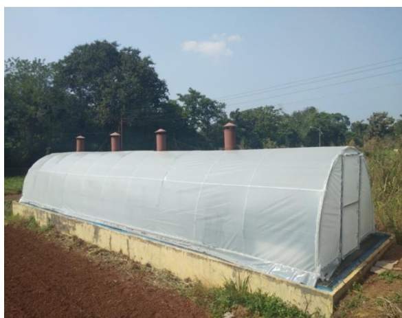
Plate 1: Outside view of Tunnel Dryer
