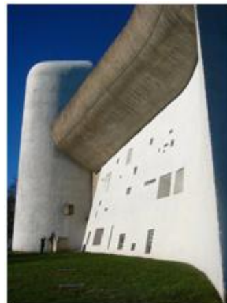
Photo 21: Neuterd de Roschamp church side perspective shows it's the curved walls Source: archdaily.com/84988
