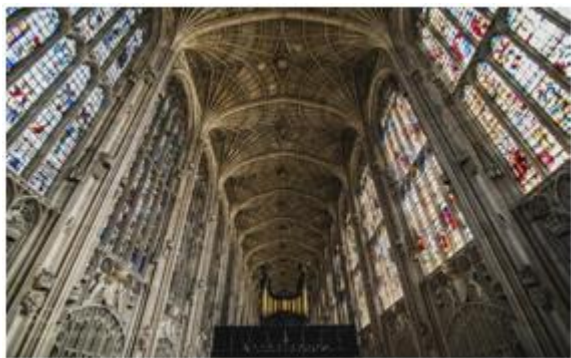
Photo 10: Shows King's College Church van vault roof structure Source: King's-College-Chapel-Cambridge-23486
