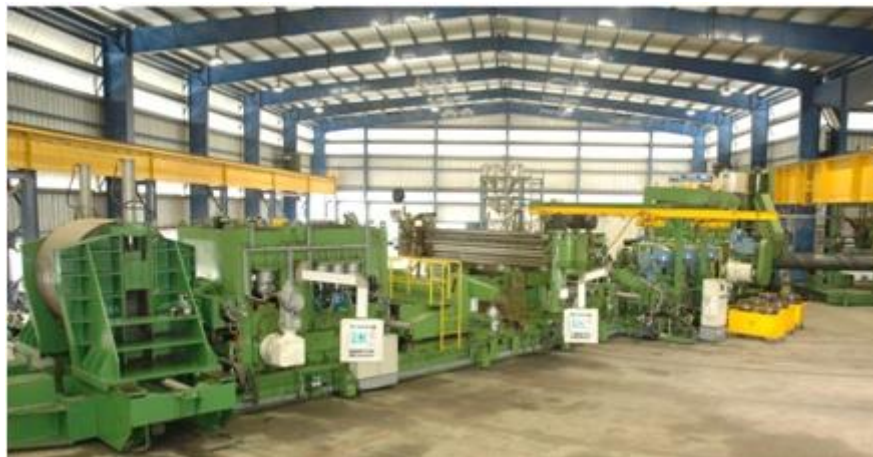
Spiral Pipemill Plant
