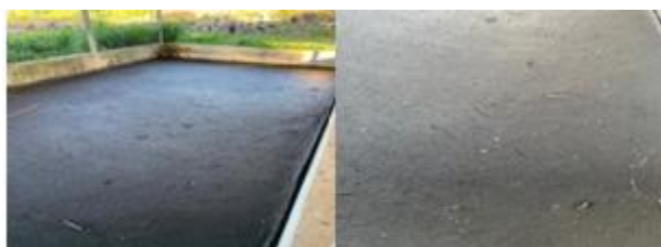
Figure 4: a) Sludge placed for dewatering; b) groove formation in the sludge after 30 days in dewatering. Paragominas, PA.
