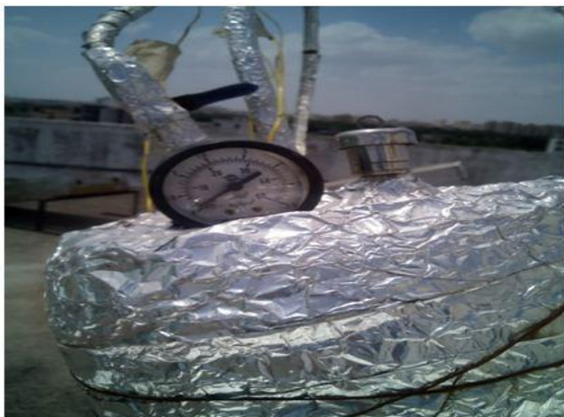
Figure 3: Copper Cylinder (Boiler)
