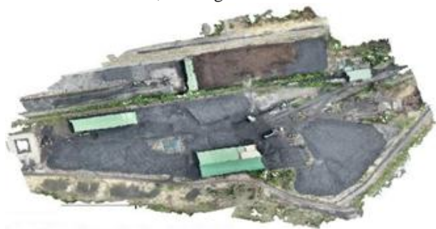
Figure 2: Point Cloud generated
