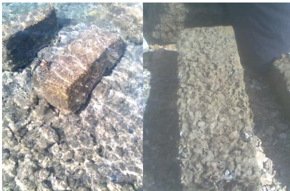
Photo 1: Submerged beam Photo(2) Submerged beam after 6 months
