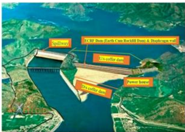
Fig 1. Photo view of location of spillway of Polavaram dam under construction across river Godavari in Andhra Pradesh in India
