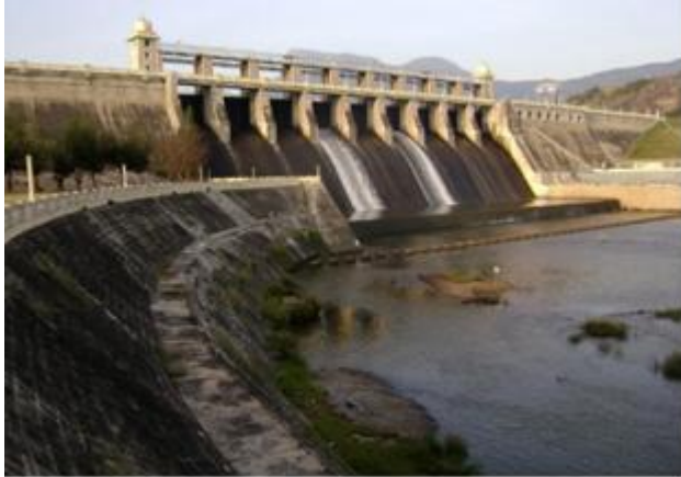
Fig 3. Photo view of an ogee spillway of Amaravati dam constructed across the River Amaravati in Tirupur district in the Indian state of Tamil Nadu
