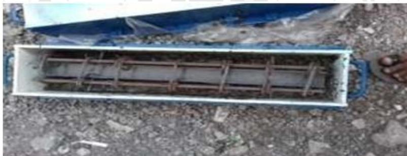
**Figure 5:** Casting of C-Channel GFRP beam
