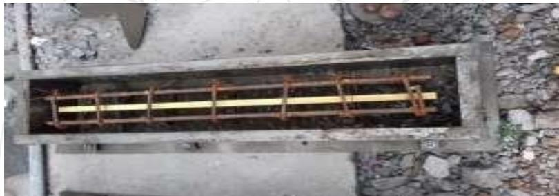
**Figure 4:** Casting of I-section GFRP beam
