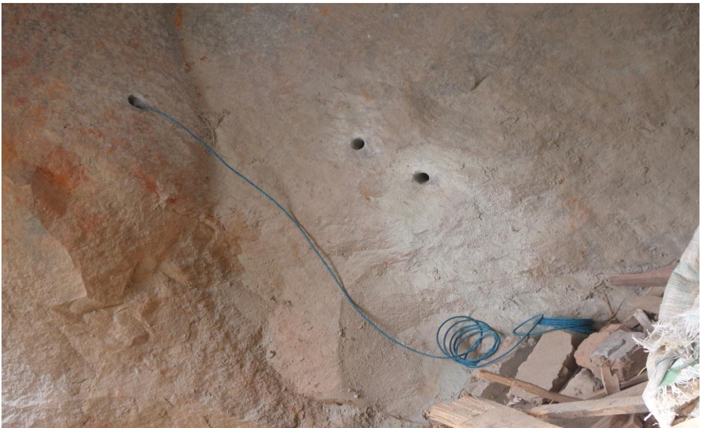
Charging of drilled holes at Gagribal Dal Lake Srinagar (Picture 02)
