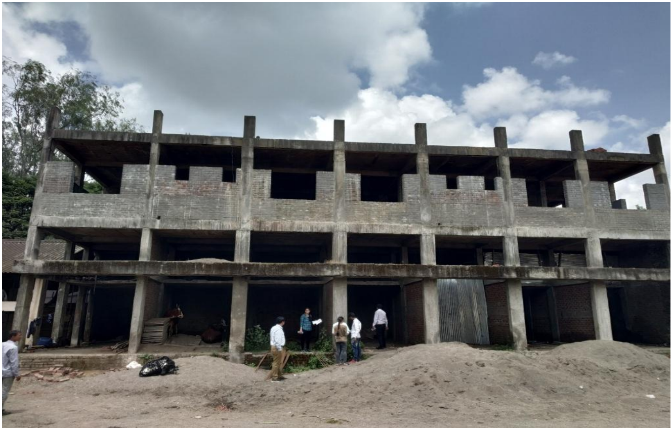
Figure 3.3: Building whose columns failed
