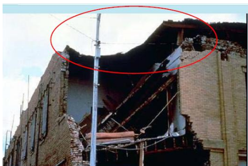
Figure 6: Weak Floor-Roof connection [6]
