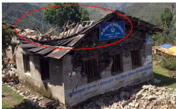
Figure 7: Weak Floor-Roof Connection [6]
