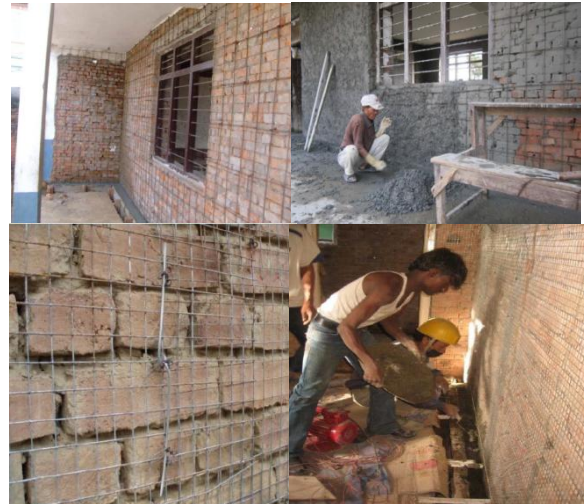
Figure 7: Steel Cage and G.I. wire mesh on masonry wall
