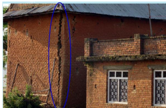
Figure 8: Connection Failure[8]
