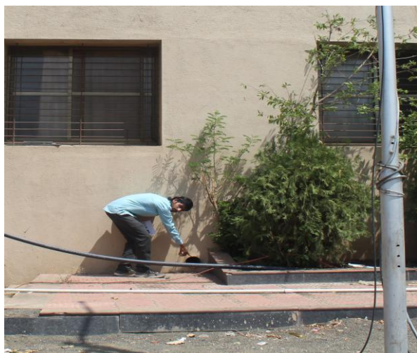
Location of 01 underground water storage tank Showing drain pipe
