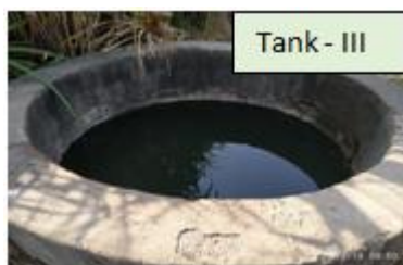
Figure: Trarabalo Hot Spring TANK 3
