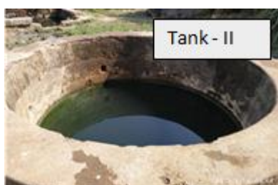
Figure: Trarabalo Hot Spring TANK 2
