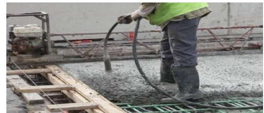
Figure 10: Concrete compaction procedure
