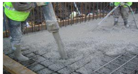
Figure 5: Concrete laying procedure
