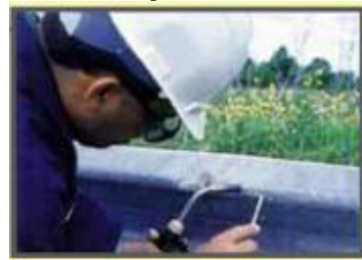
Figure 5: Zinc-Based Solder Technique
