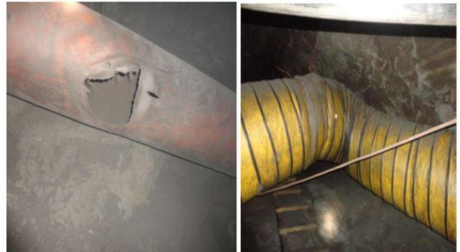
Figure 1: Air leakages and shock losses as observed at TML.
