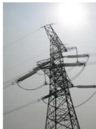
Figure 1: A 500KV tower
