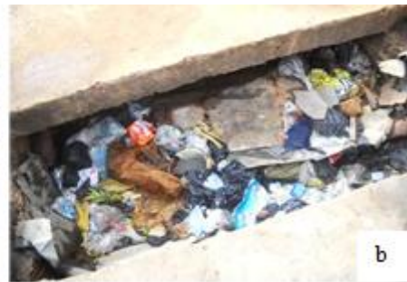
Plate 1: Open culverts filled with waste in Dèkounbé in the district of Godomey (a) and in the district of Abomey-Calavi (b)
