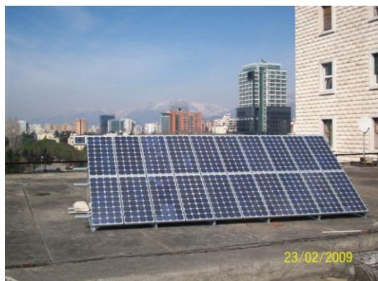
Figure 1: 1500Wp Photovoltaic panel
