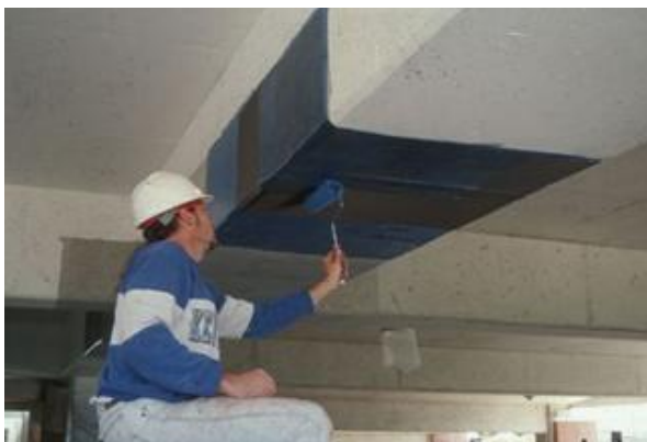
Figure 14: Concrete strengthening by carbon fibers[95]
