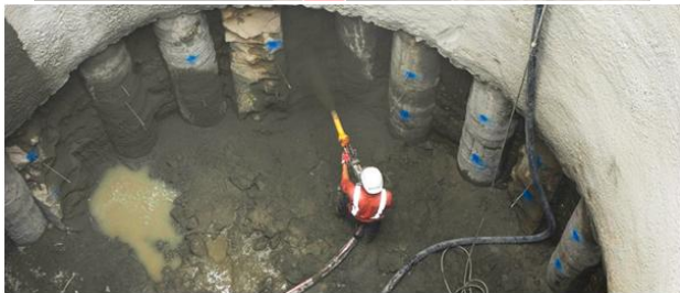
Figure 14: Fiber Reinforced Shotcrete in underground structures[94]
