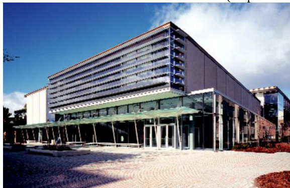
Figure 24: York University - computer science building. (Courtesy www.pkphotography.com)
