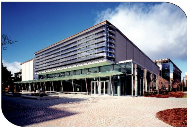
Figure 24: York University - computer science building. (Courtesy www.pkphotography.com)
