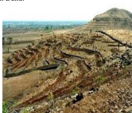
Figure 4: CCT in Hiware bazar
