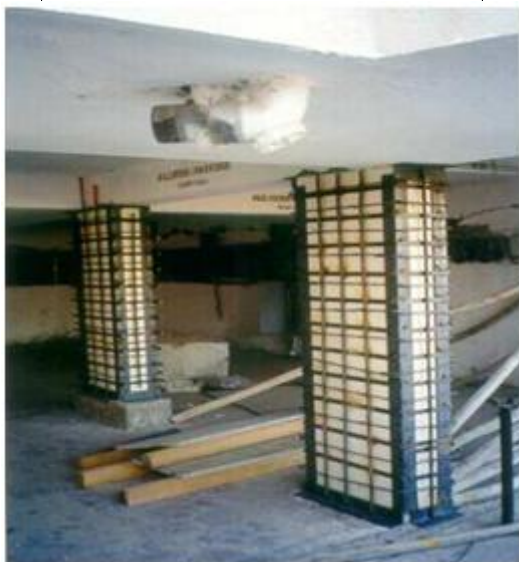
Figure 5: Steel Jacketing of column
