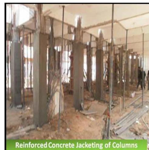
Figure 4: Jacketing of Column (Source MRB & Associates)
