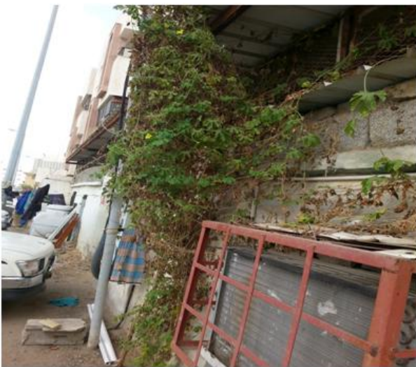
Figure 7: Vine impact to Building and Structures
