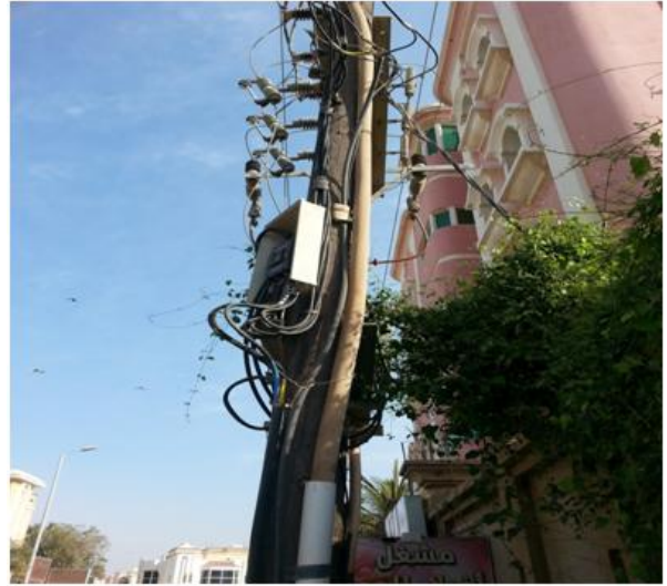
Figure 8: Vine impact to Electric Transformer
