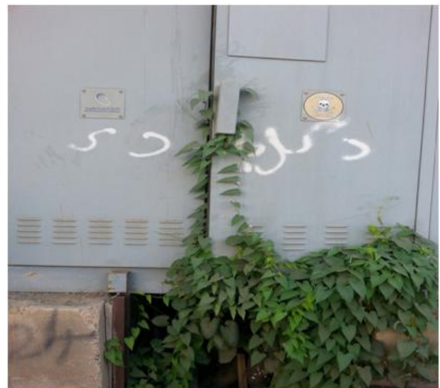
Figure 9: Vine impact to Volt Cabinet
