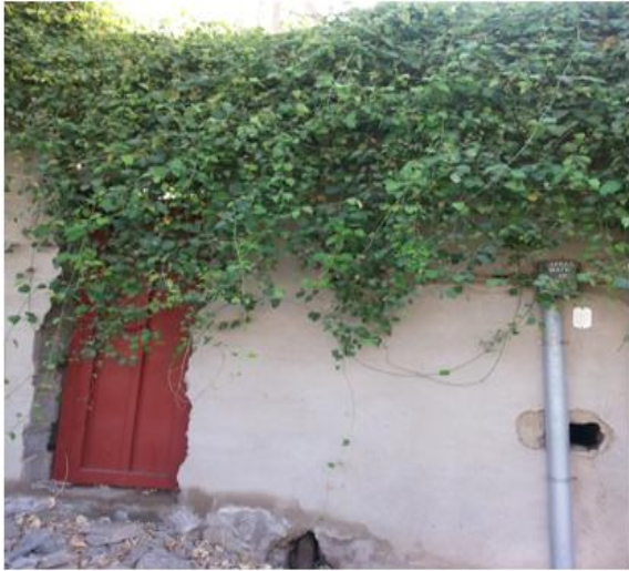
Figure 6: Vine impact to Fence and Door Recreation
