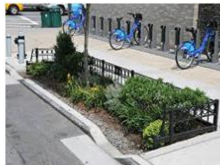
Figure 5: Bioswales along the curb-side
