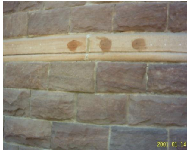
Photo 10: UPV Test Jodhpur A&M Office
