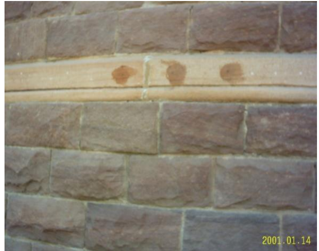
Photo 10: UPV Test Jodhpur A&M Office
