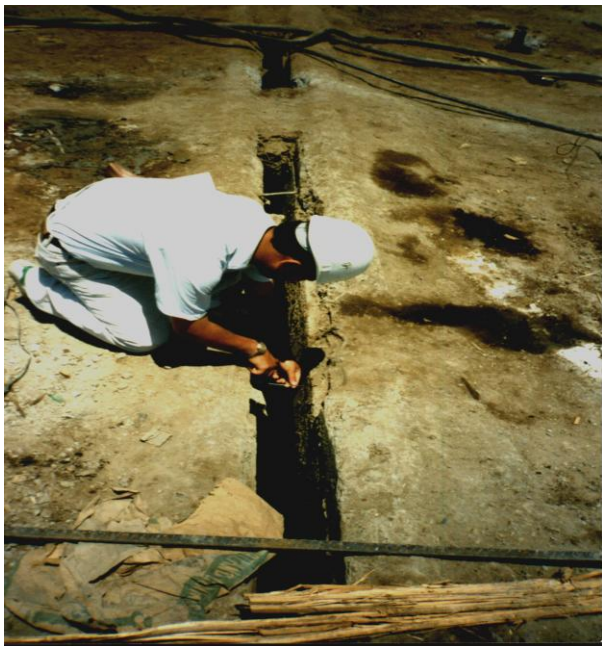
Figure 4: Wide gap due to differential settlement in Damietta bridge
