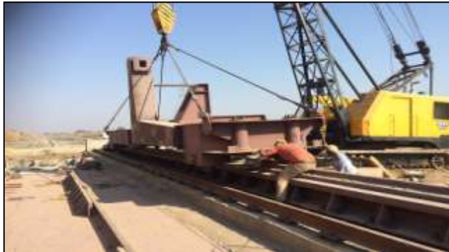
Figure 13: Erection of the Side arm charger
