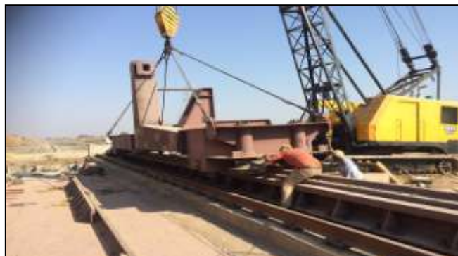
Figure 13: Erection of the Side arm charger
