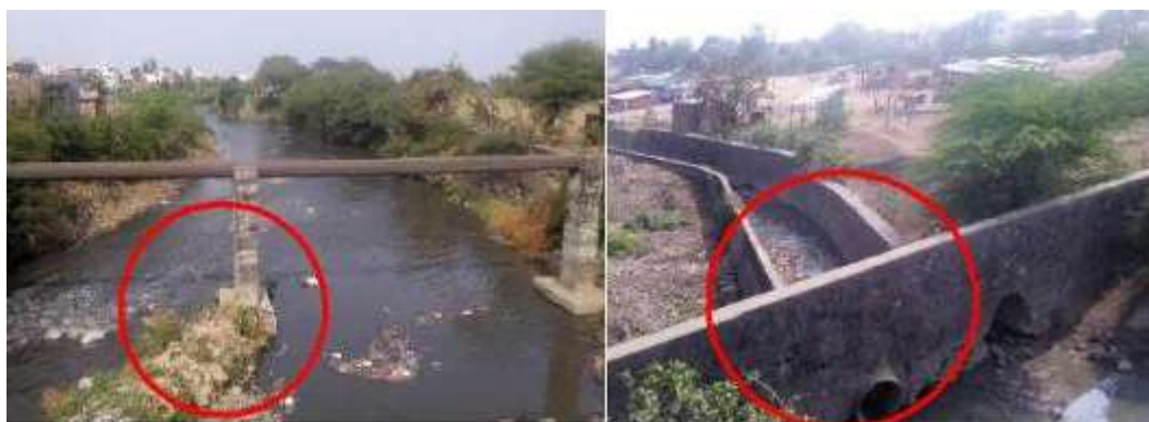
Figure 20: River channel near Jagnade Chowk
