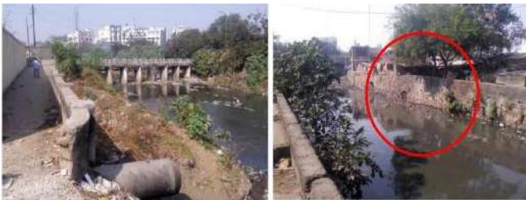
Figure 16: River channel near Buldi bridge
