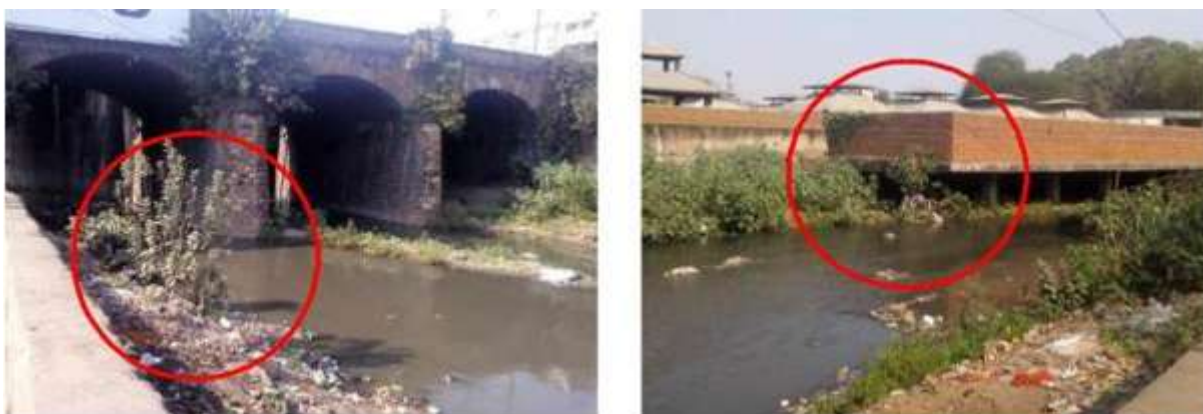
Figure 17: River channel at Mokshadham (Crematorium)
