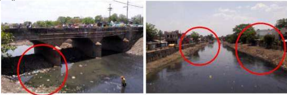
Figure 19: Tulsi Bagh bridge – Nag river
