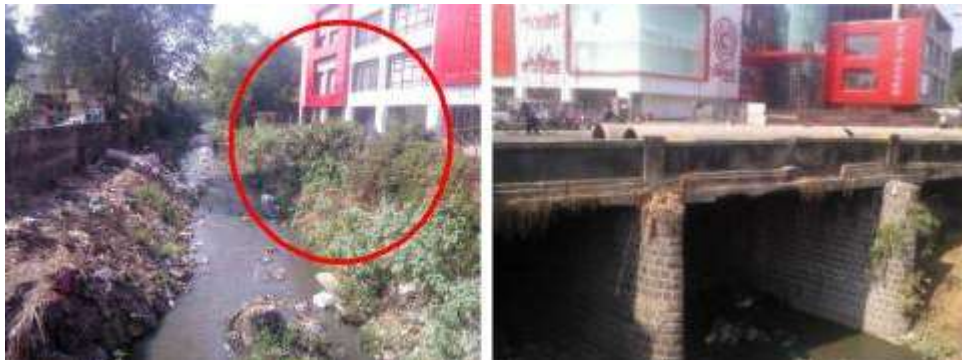
Figure 13: River channel at Central Mall
