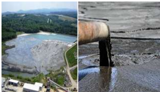
Figure 1: Storage Lagoons of Pond Ash
