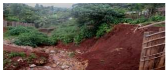
Figure 1: Rills caused by land use change In Melka Hola
