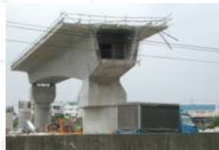
Figure 1.1: Box Girder Bridge
