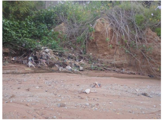
(Plate 4). Gully erosion in Barunde
