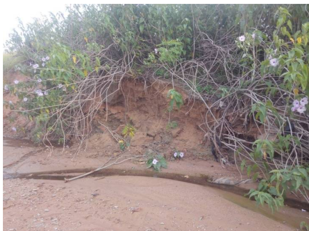
(Plate 7). Gully erosion in M/INNA.
